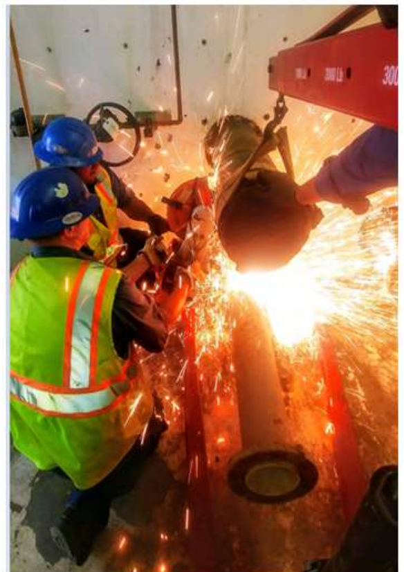
Water Operators Cutting Ductile Iron Pipe.
